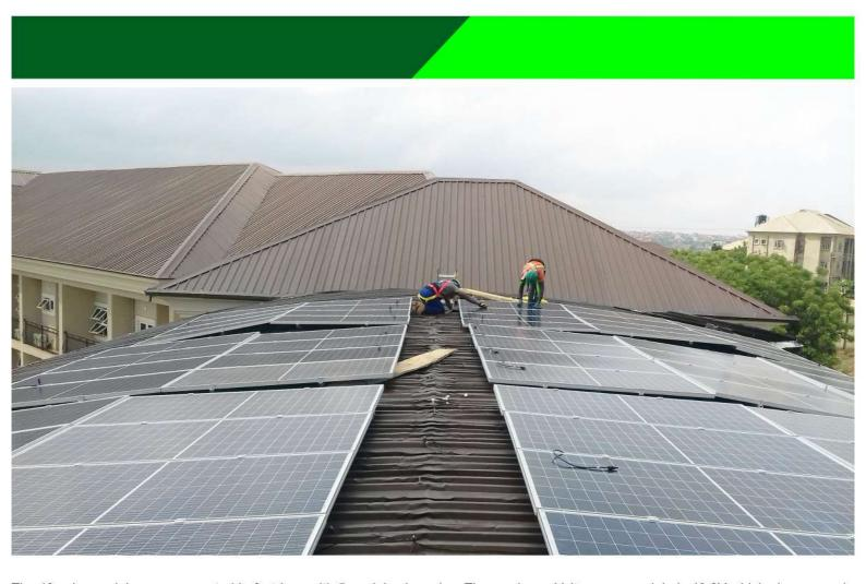
The 40 solar modules are connected in 8 strings with 5 modules in series. The maximum Voltage per module is 43.2V which gives a maximum voltage (STC) of 5 x 43.2V = 216V. Since the temperature in Lagos is never below  $25^{\circ}$ C (STC), the maximum Voltage will be always less than the allowed 250V of the charge controller.
